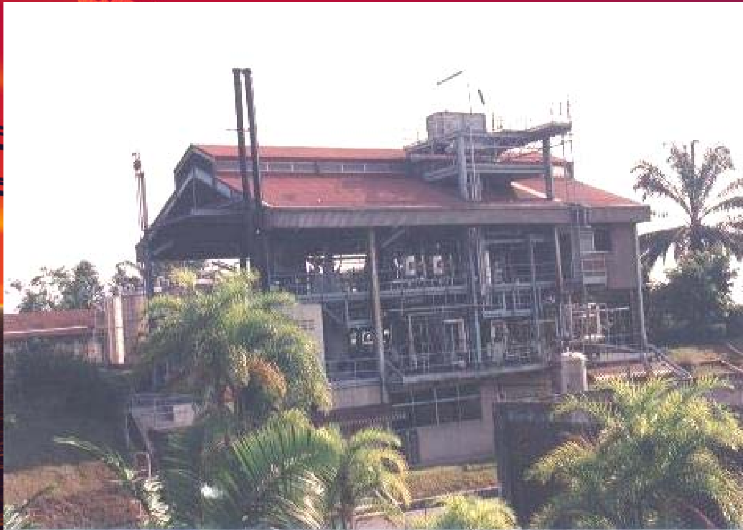
Palm Diesel Pilot Plant at MPOB (3,000 tonnes per year)
